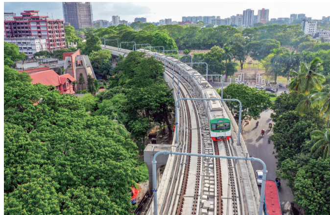
The MRT 6 rapid transit line of the Dhaka Metro Rail
